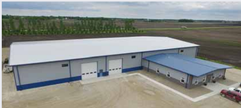
The company quickly outgrew its 12,000-square-foot shop and built this 27,000-square-foot shop in 2014. They are now outgrowing it. RUSH RIVER STEEL PHOTO
