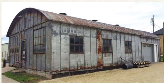
Trachte Brothers Co. was one of the earliest companies in the U.S. to use stationary roll formers. Originally located in Watertown, Wisconsin, its first roll former was used to make corrugated water tanks for livestock. A second part of the business included metal barrel-vaulted buildings made with 2' wide roll-formed corrugated panels. Early Trachte buildings, like this one in Brodhead, can still be found in the Madison, Wisconsin area. PHOTO COURTESY OF TRACHTE BUILDING SYSTEMS
