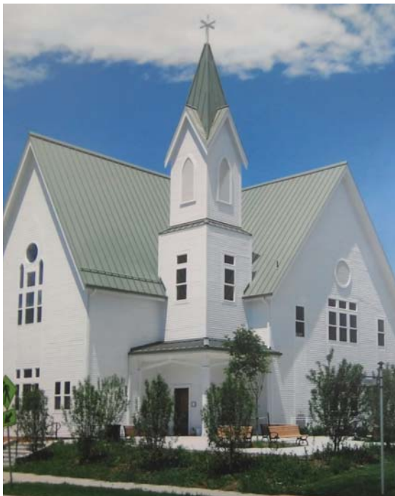
This church in Broomfield, Colorado, is one of many roofing jobs roll formed and installed by Orsborn.
