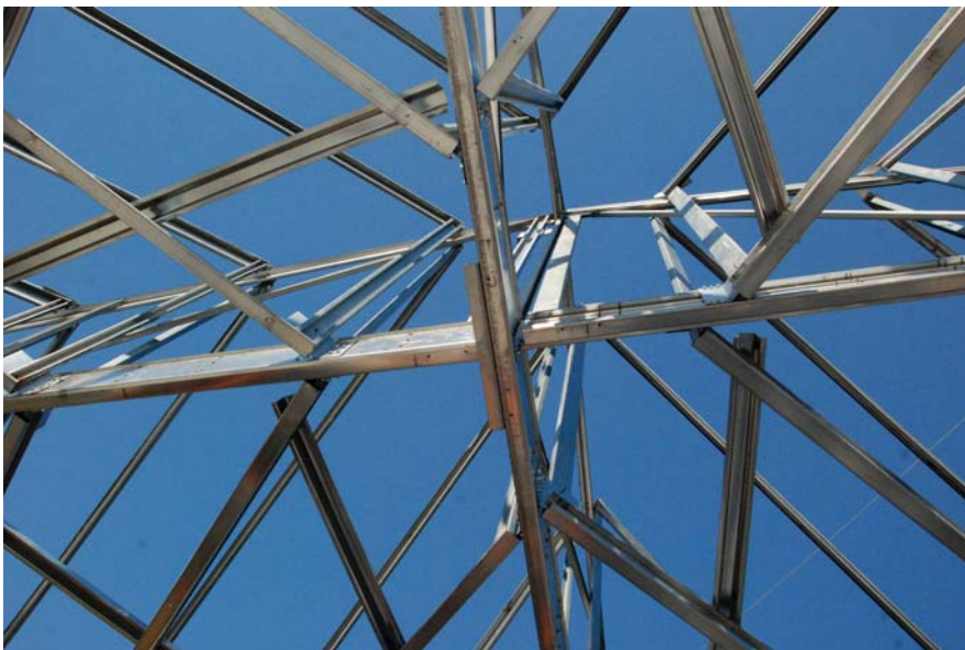
LGS/CFS roof trusses. Photo courtesy of SFIA
