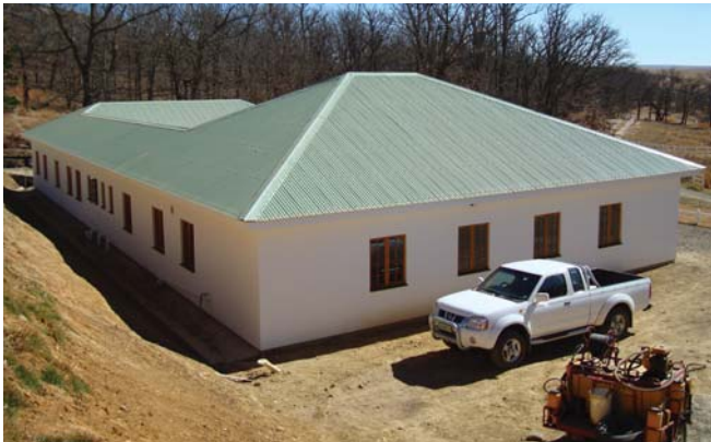
CFS is more common in overseas countries. These before and after photos are from a building project in South Africa: a polo club and farm stay called Oaklands Farm Stay . Photos courtesy of Howick Ltd.
