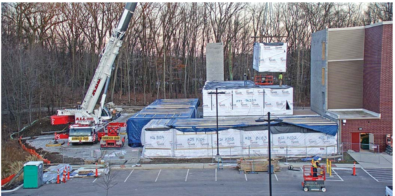
ToVee modular units being craned into place. They were being used to create an addition to an existing building. Photo courtesy of ToVee
