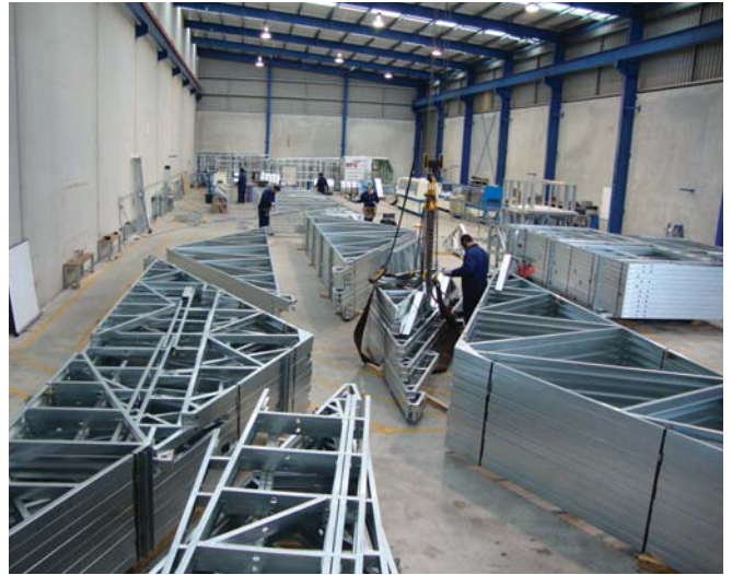
Roof trusses production at Rollforming Services, Auckland, New Zealand. Photo courtesy of Howick Ltd.
