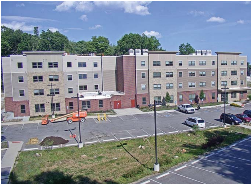
Once in place, the modular units blend with the existing building design. Photo courtesy of ToVee
