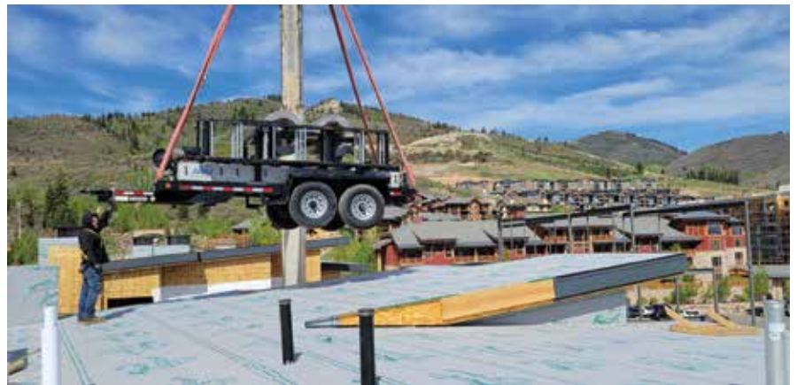
If needing to lift your machine to roof height you’ll want an open flatbed like this Maxey Trailer owned by Homie Mulcahy of SaltedMetals in Utah. Note that when the roll-forming trailer is lowered, it will be jacked and stabilized to hover just over the roof so as not to put extra weight on the roof structure. PHOTO COURTESY OF SALTEDMETALS ARCHITECTURAL METALS DESIGN AND CONSULTING
