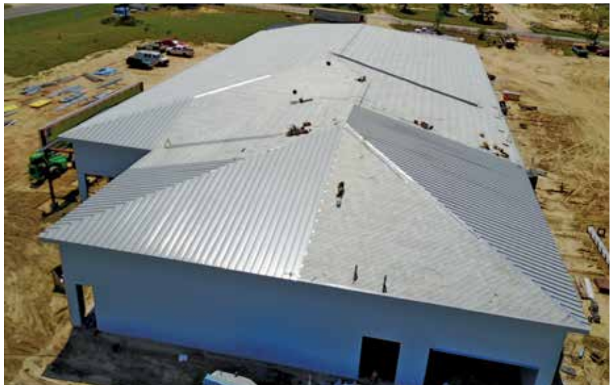
ABOVE: Dune Lakes Elementary School, Walton County, Florida: 163,200 sq. ft. Englert 2400 Series Standing Seam Roof (.032 aluminum Dove Gray Kynar Finish).
