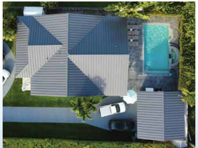
Residential home, Doral, Florida, Coastal Metal ML-150, 1.5", 24 ga. Galvalume, Charcoal Gray. PHOTO COURTESY COASTAL METAL ROOFING SALES.
