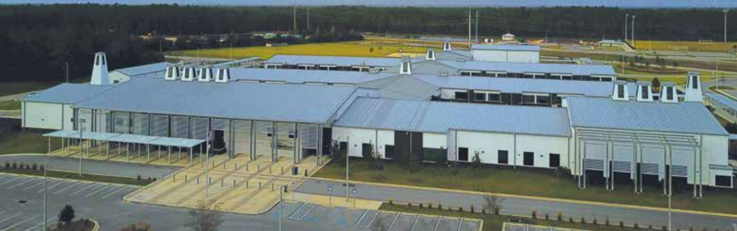
ABOVE: Dune Lakes Elementary School, Walton County, Florida: 163,200 sq. ft. Englert 2400 Series Standing Seam Roof (.032 aluminum Dove Gray Kynar Finish).
