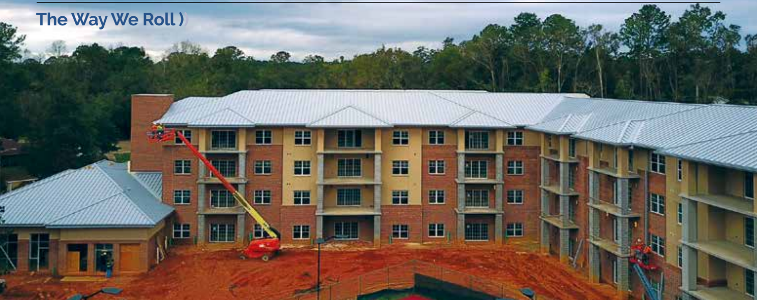
West Minister Oaks Retirement Village, Tallahassee, Florida: 27,300 sq. ft. Petersen Tite-Loc Plus Standing Seam Roof (24 ga. Cityscape Kynar Finish), 7,000 sq. ft. Fibertite single-ply roof. PHOTOS COURTESY KENT CONSTRUCTION AND ROOFING, INC.
