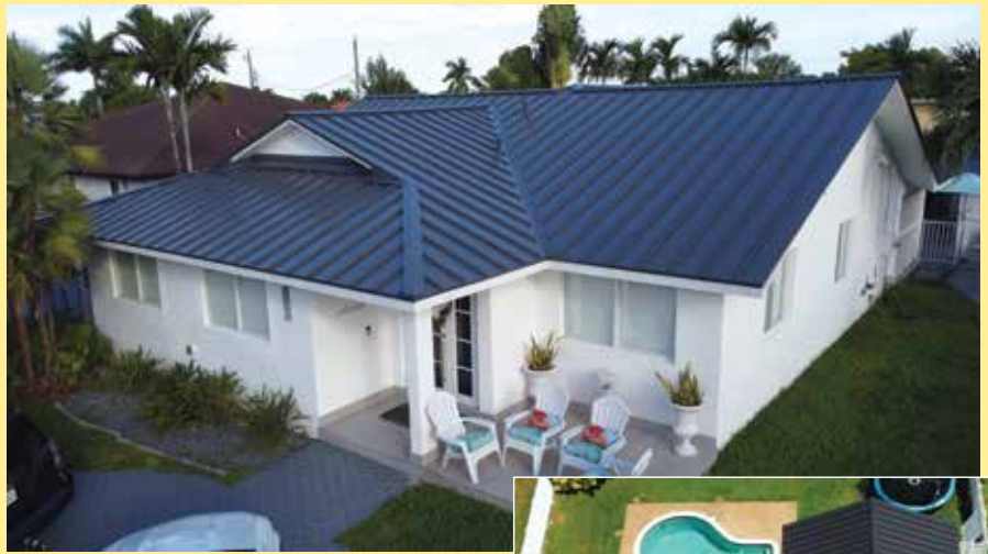
ABOVE: Residential home, Doral, Florida, 24 ga. Coastal Metal Mechanical Lock, 1.5", Charcoal Gray. RIGHT: Residential home, Davie, Florida, 24 ga. Coastal Metal Mechanical Lock, 1.5", Midnight Bronze. PHOTOS COURTESY COASTAL METAL ROOFING SALES.
