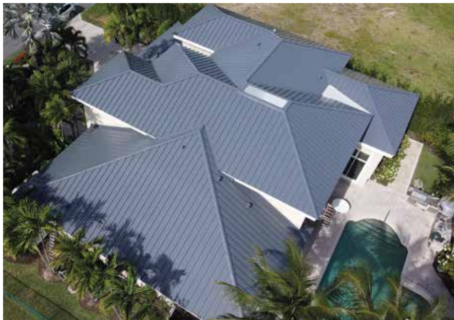
Residential home, Hallandale Beach, Florida, Coastal Metal Mechanical Lock, 1.5" (0.032 aluminum) Charcoal Gray. PHOTOS COURTESY COASTAL METAL ROOFING SALES.
