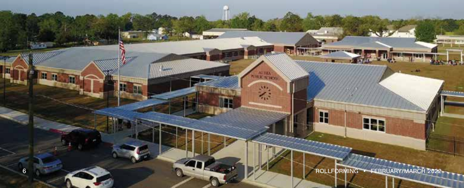
BELOW: Altha Public School, Altha, Florida: 136,997 sq. ft. Englert 2400 Series Standing Seam Roof (24 ga. Galvalum Finish). PHOTO COURTESY KENT CONSTRUCTION AND ROOFING, INC.
