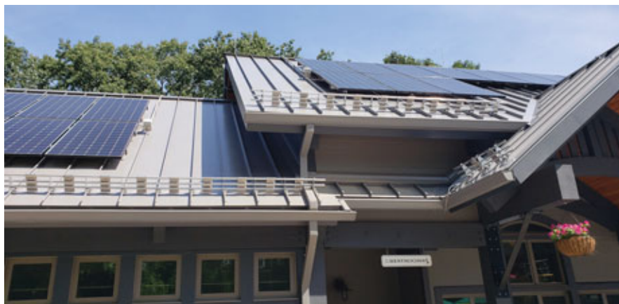
Metal roof clamps with a patented, non-penetrating sliding-pin design from AceClamp secure these solar arrays and snow retention systems. PHOTO COURTESY OF ACECLAMP.
