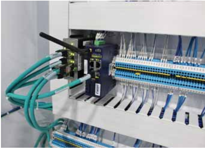
The typical EWON unit is located inside the Motor Control Center of a roll-forming line. ASC MACHINE PHOTO
