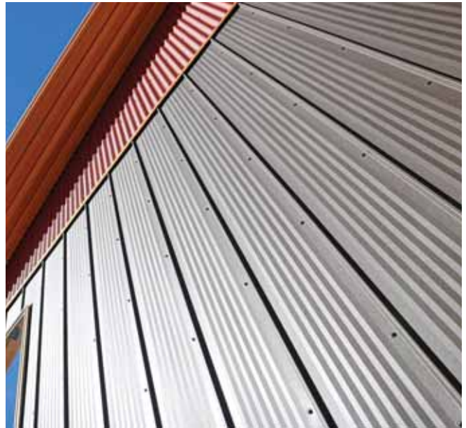
A close-up view of an installed board and batten panel. MRS PHOTO
