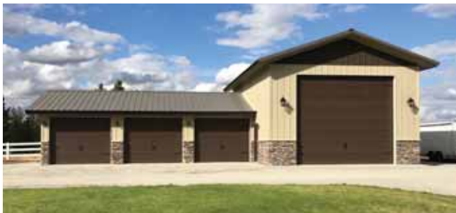
A building with quad rib panel. MRS PHOTO
