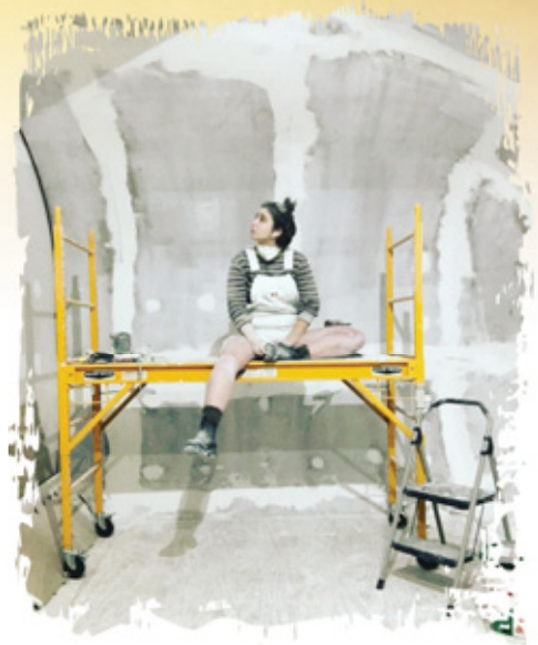
Nolee Anderson, trim carpenter
