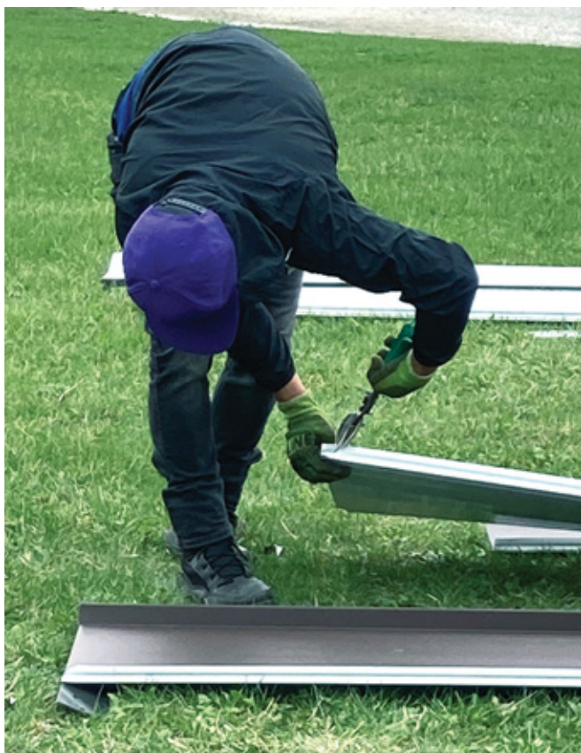
A crew member notching panel for fitting.
