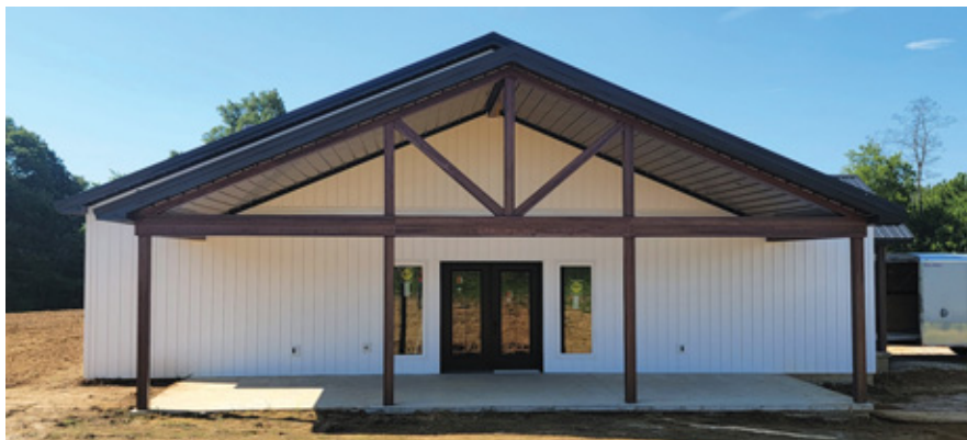
This building features white board and batten wall panel plus the use of the new Tru>Metal HD digital paint panel from Steel Dynamics on the beams of the front façade. GRABER POST PHOTO
