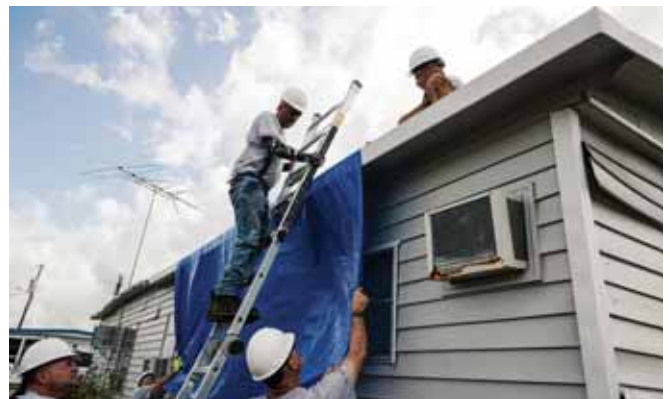
Hurricane response in Florida.
