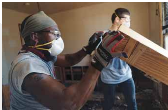
Rebuilding in Selma, Alabama.
