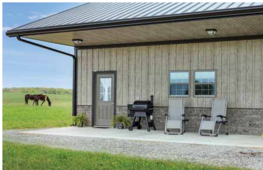
In addition to a standing-seam metal roof, this building features metal board and batten siding that looks like wood and steel wainscot that looks like stacked stone. PHOTO COURTESY OF LITTLE HARVEYS.
