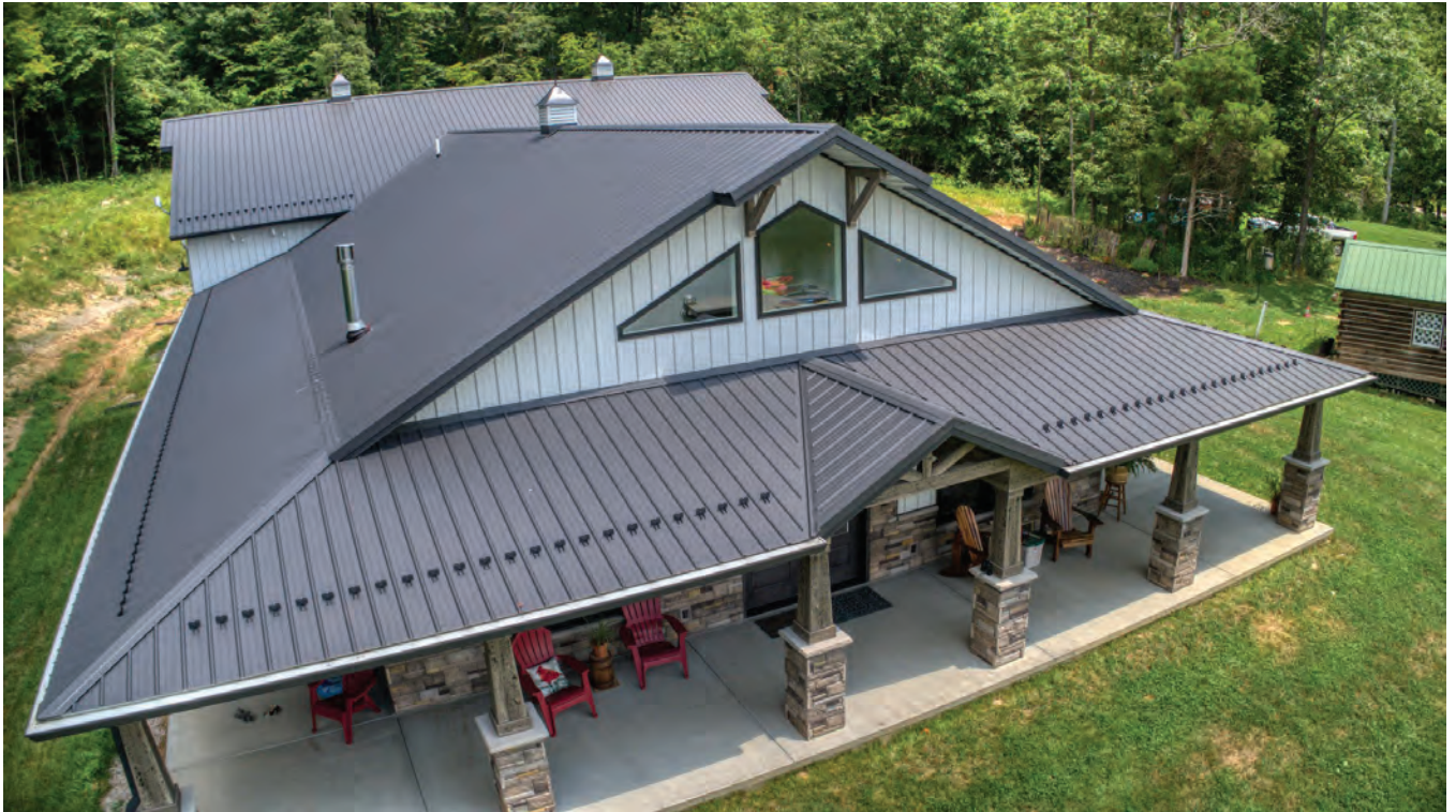
Metal roof featuring AkzoNobel's CERAM-A-STAR® Select Frost. PHOTO COURTESY OF GRABER POST BUILDINGS.
