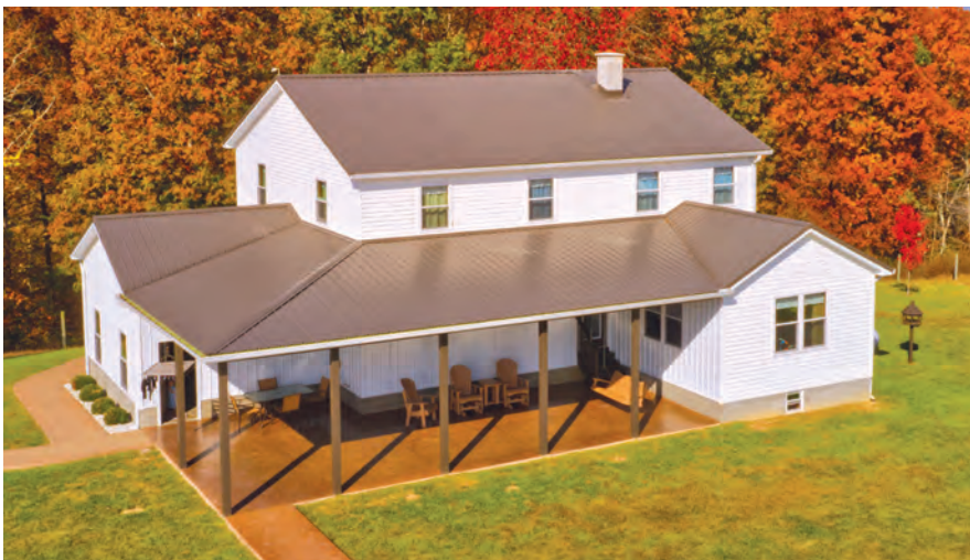
Barndominium built with Progressive Metals Coil
