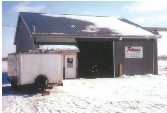
Ramco's original facility.
