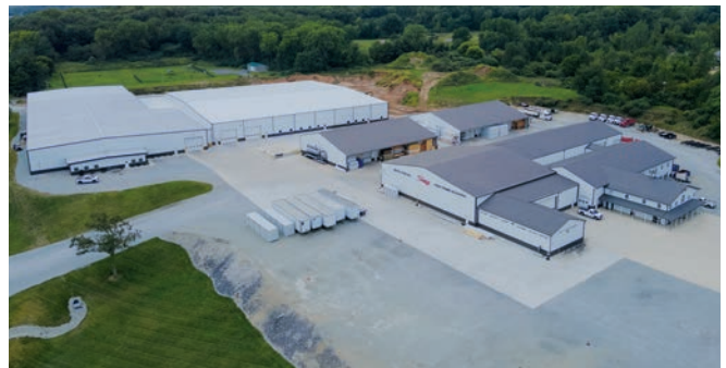
The Rochester, Indiana, facility.
