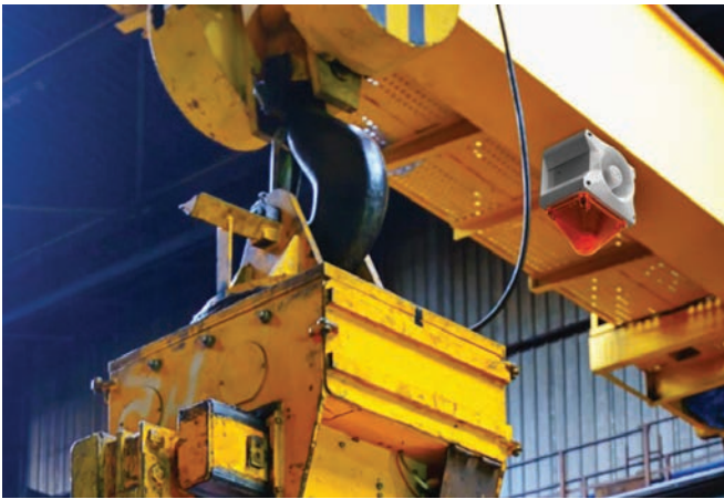
When looking to maximize safety in environments with overhead cranes, dual sounder and strobe combination signaling devices are especially recommended.
