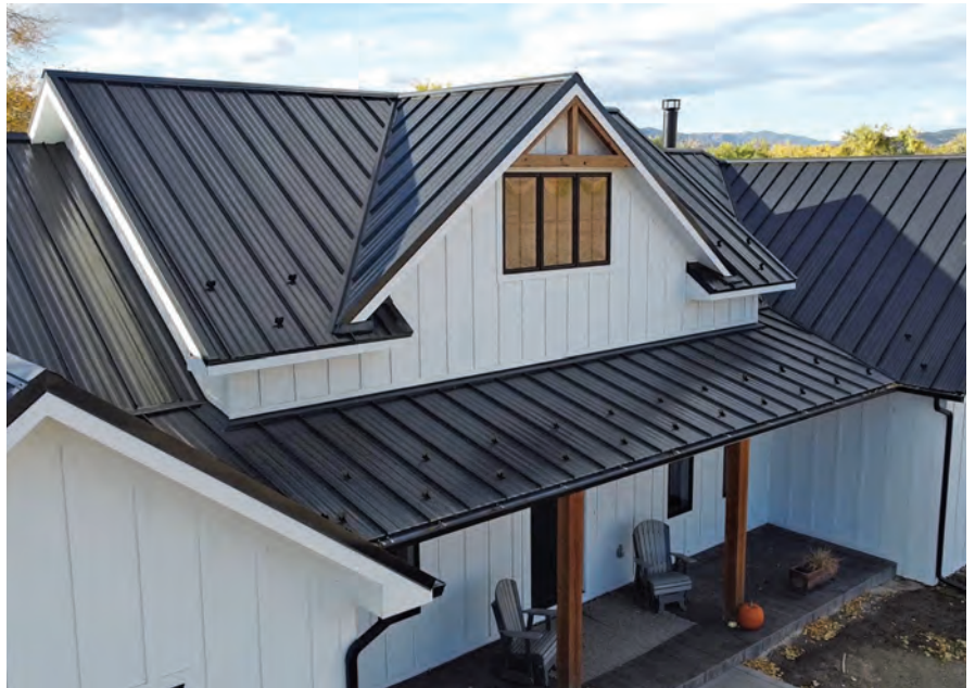
Photos tell stories and improve trust and credibility in a product. Roofing project completed with Legacy Metal Center Metal Panels. COURTESY OF LEGACY METAL CENTER
