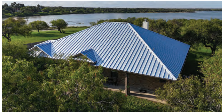
A grey standing seam metal roof installed by South Texas Metal Roofing. COURTESY OF THE METAL ROOFING ALLIANCE.
