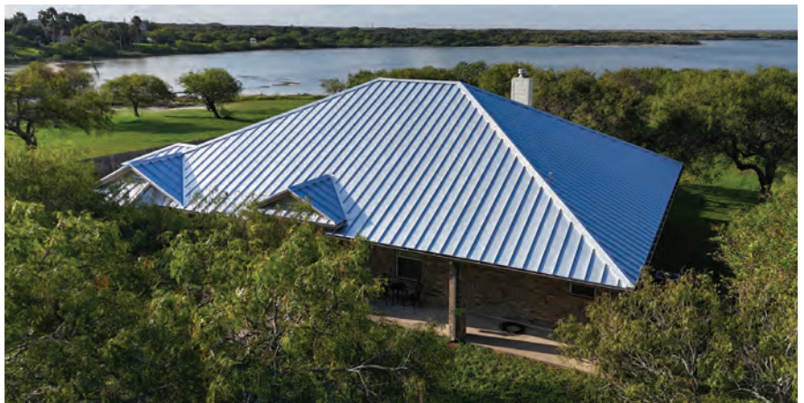
A grey standing seam metal roof installed by South Texas Metal Roofing. COURTESY OF THE METAL ROOFING ALLIANCE.
