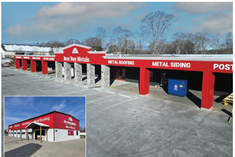
The latest expansion in Greer/Greenville, South Carolina, brings a major upgrade to the Best Buy Metals Eastern Region with enhanced production, showroom, and customer service capabilities. INSET: The Dalton, Georgia, store represents an important milestone in the company's expansion and commitment to contractor support.
