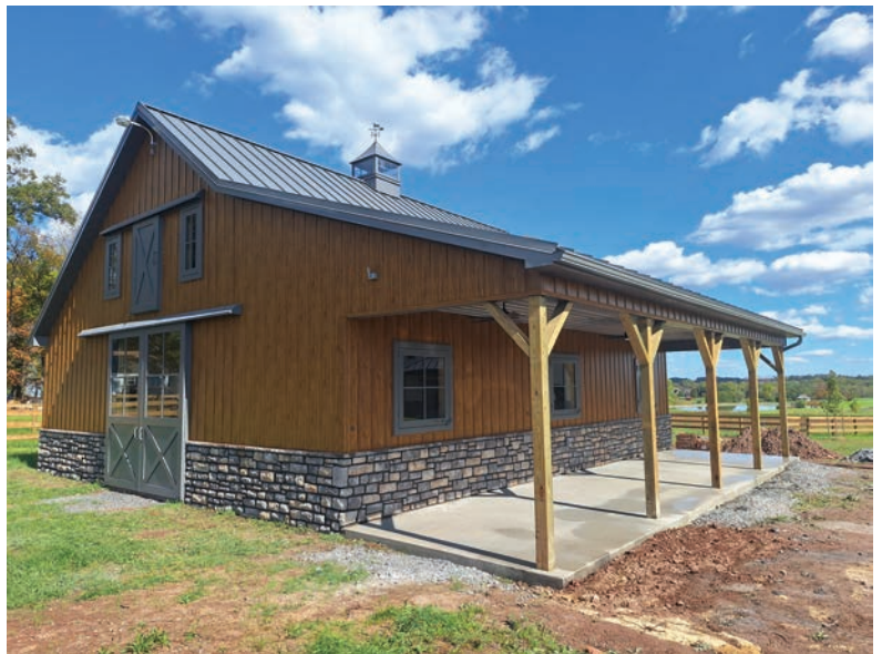
Board and batten siding has experienced a surge in interest in recent years.
