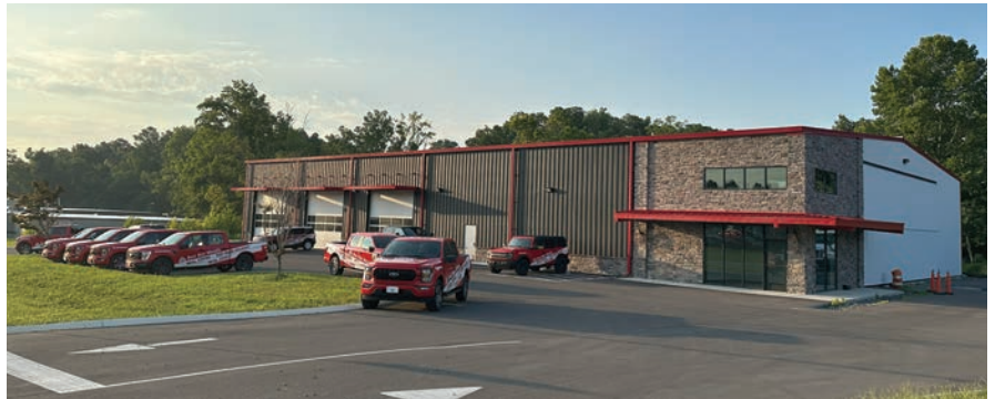
This new warehouse and production facility at the Cleveland, Tennessee, location serves as a key hub and enhances already streamlined operations and efficient service. PHOTOS COURTESY OF BEST BUY METALS.
