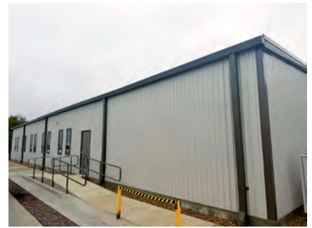
To support continued growth within its Engineering and Mechanical Customer Service Departments, Bradbury has expanded its customer service workspace to 3,000 square feet, up from approximately 1,700 square feet. Photo courtesy of Bradbury.
