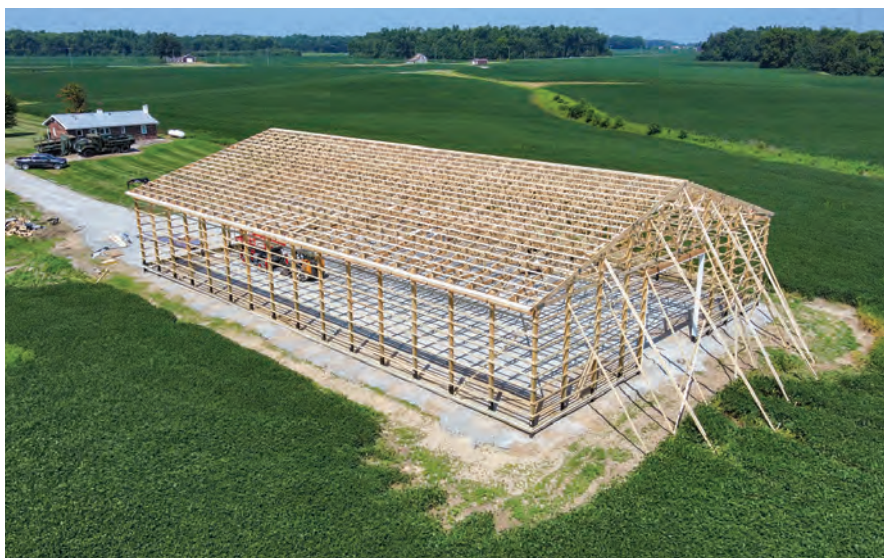
An agricultural post-frame building going up.
